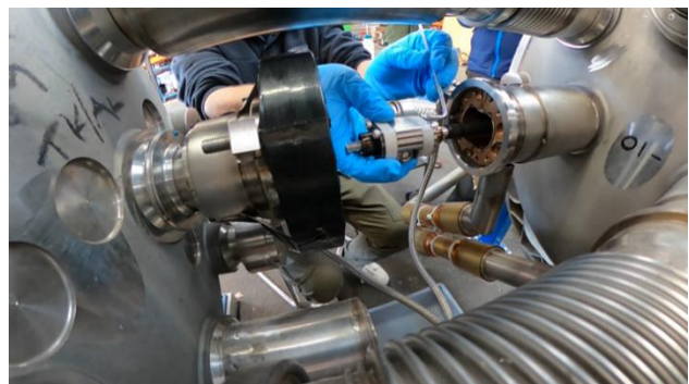
Figure 2: On-going assembly of the coating train (central part) in the beam screen, within a magnet interconnection.
