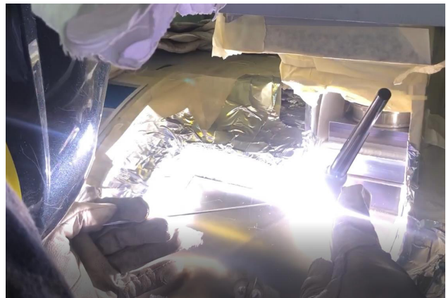
Figure 10: Aluminium tank TIG welding.
