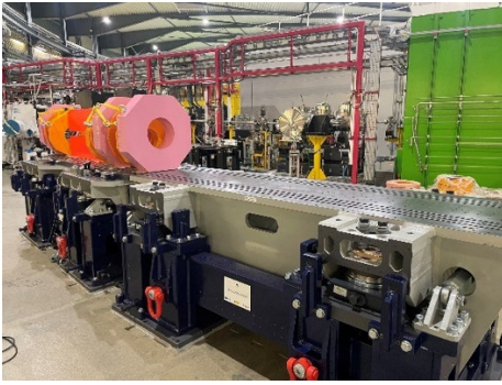
Figure 6: Girders prototypes installed at the Experimental Hall of ALBA, being tested.
