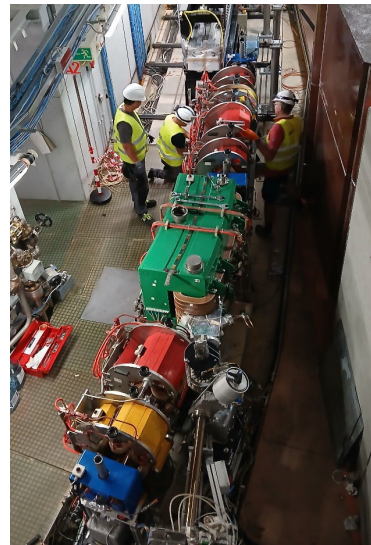
Figure 2: View of the SR (roof removed).
