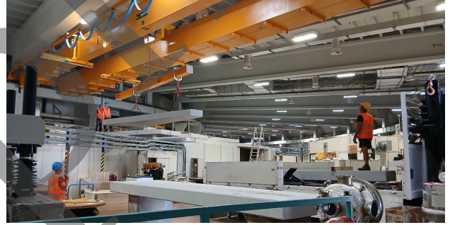
Figure 1: Slabs removal from SR roof.
