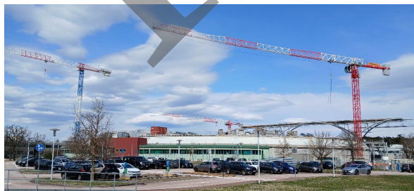
Figure 8: Cranes around the Main Building of Elettra.
