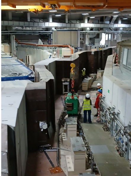
Figure 3: Removal of the last magnet from SR.
