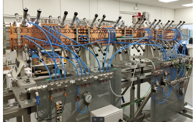
Figure 1: ESS-Bilbao RFQ connected to the cooling skid during the first water-cooling and frequency characterization campaign.
