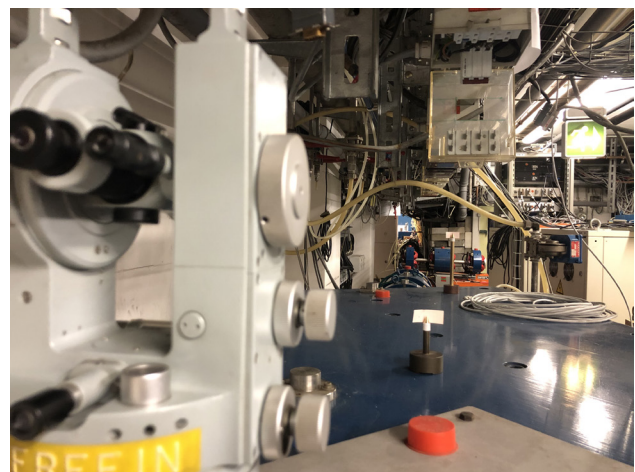
Figure 2: Optical alignment of the dipoles and triplets using theodolites.
