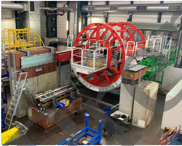
Figure 6: E2 during insertion test at 90degrees.
