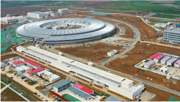
Figure 1: Hefei Advanced Light Facility (HALF) currently under construction in Hefei, China.
