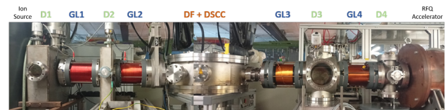
Figure 7: Low energy beam transport channel at Goethe University (GL – Gabor Lens, D – Diagnostic chamber, DF+DSCC – Deflector and De-compensator).
