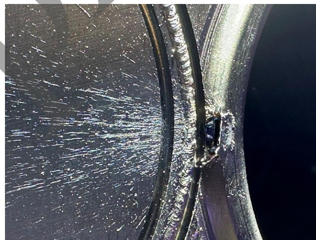
Figure 5: Pin hole breach of the vacuum flange for the beam absorber.
