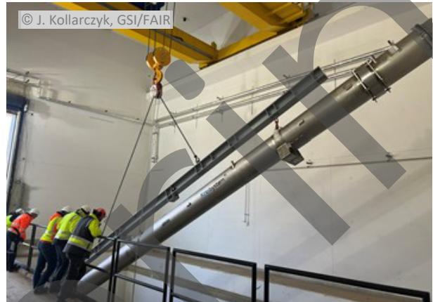
Figure 12: Lifting of a 13 m long section of the cryogenic bypass line connecting the cryogenic components across the warm sections.
