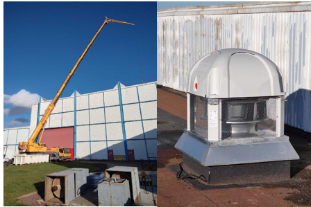
Figure 6: Installation of the new air extraction towers.
