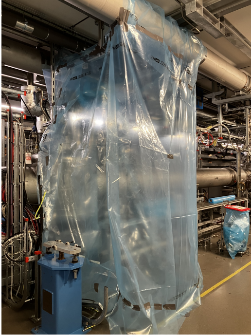
Figure 2: LWUs and dummy pipes removed. Booth when preparing VB piping.
