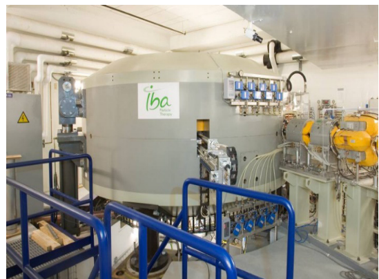
Figure 2: IBA 230 MeV resistive isochronous cyclotron [7].
