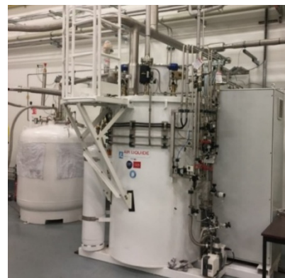
Figure 7: S3 Cold Box (Helial SF from ALAT).
