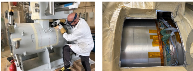
Figure 15: repairing LTS wire inside a SMT.
