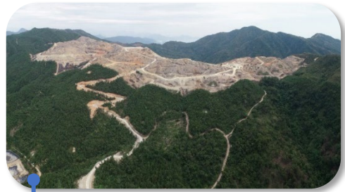
Civil construction began
