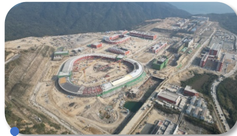
Testing Auxiliary system
