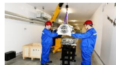
June 28, 2021 HEPS Installs First Piece of Accelerator Equipment in Linac Tunnel.
