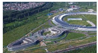
Nov. 3, 2023 Civil Construction for ancillary buildings completed
