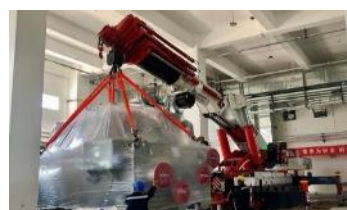
Apr. 13, 2021 Utility installation in NO.2 Hall commenced
