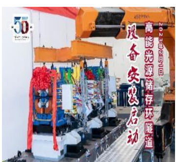
Feb. 1, 2023 The first girder was installed in the storage ring tunnel
