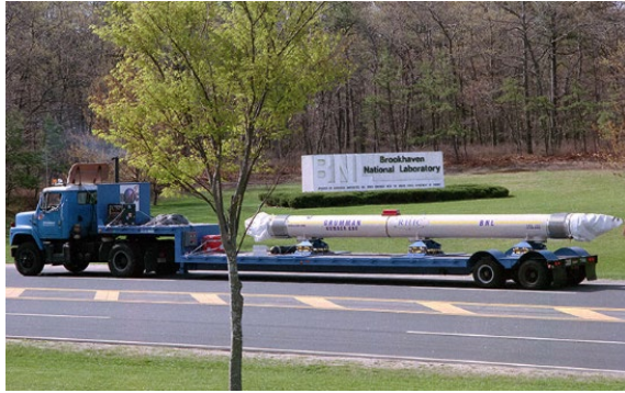
collider installation begins
