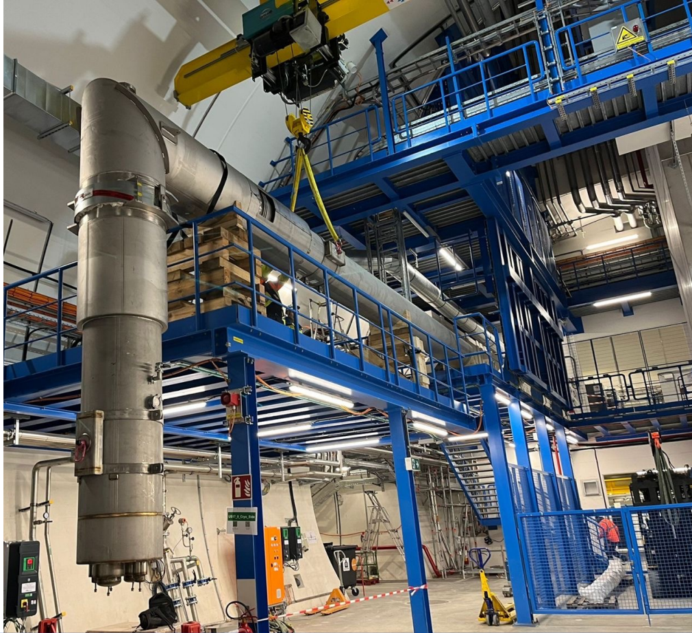
Lowering and temporary storage of first spools for connection to QPLG in Pt5
