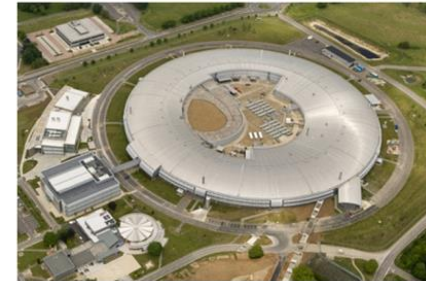
Diamond (2007) 3 GeV \epsilon_x = 3.0 \text{ nm} , \epsilon_y = 30 \text{ pm} , I = 300(500) \text{ mA}
