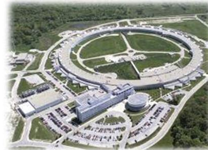
APS (1995) 7 GeV \epsilon_x = 2.5/3 \text{ nm} , \epsilon_y = 30 \text{ pm} , I = 100 \text{ mA}
