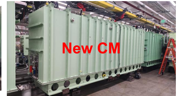
First cryomodule replacement in linac tunnel (Summer 2024)
