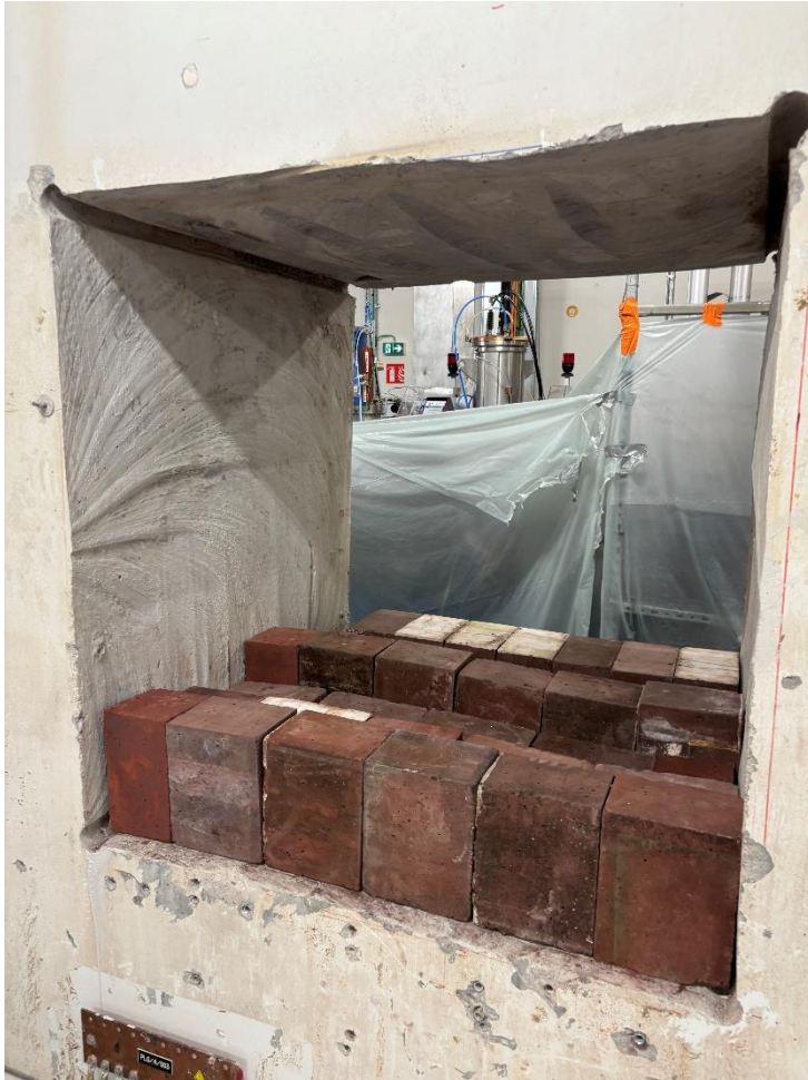
Drilling through the SPIRAL2 wall for the NEWGAIN beamline
