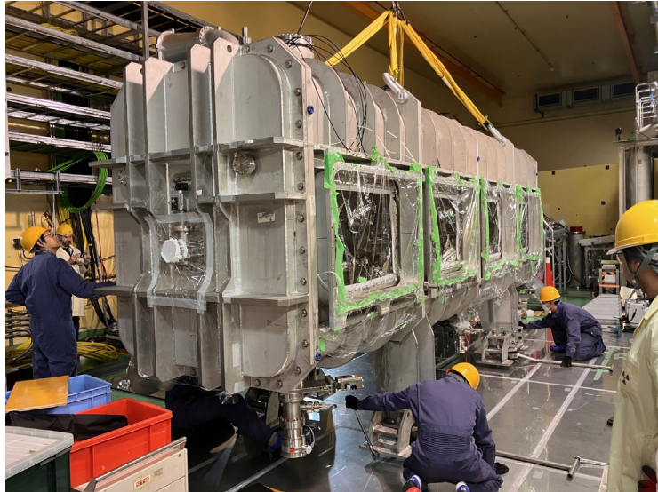
Installation to the beam line
