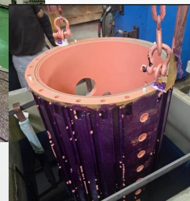
DTL tank fabrication (machining and Cu-plating)
