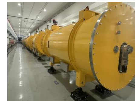
Installation completed to CM062
